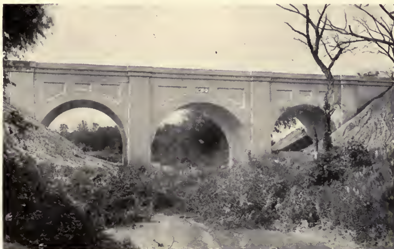
VANDALIA RAILROAD. CONCRETE BRIDGE OVER SALT CREEK, EAST OF EFFINGHAM ON LINE OF OLD NATIONAL ROAD
